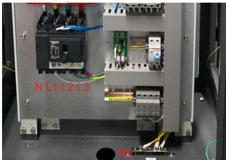
Figure 1 - Main Breakers
