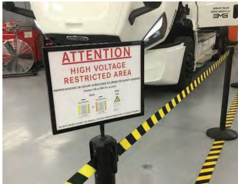
Electrical Safety Area
